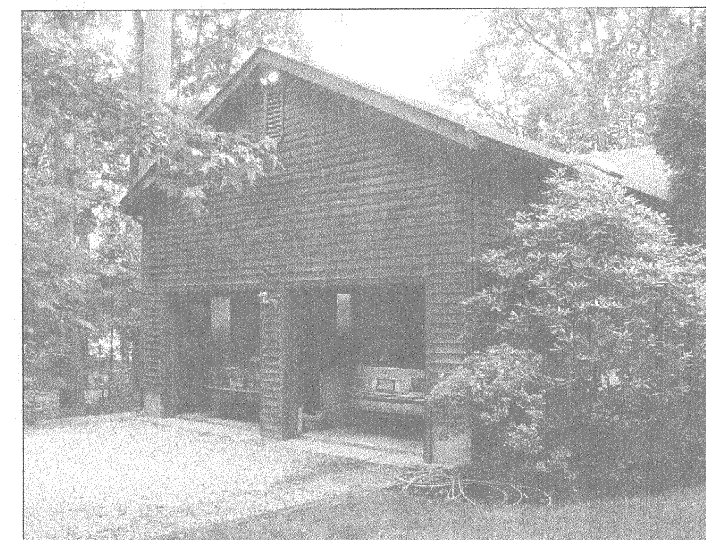
RIGHT SIDE - GARAGE
